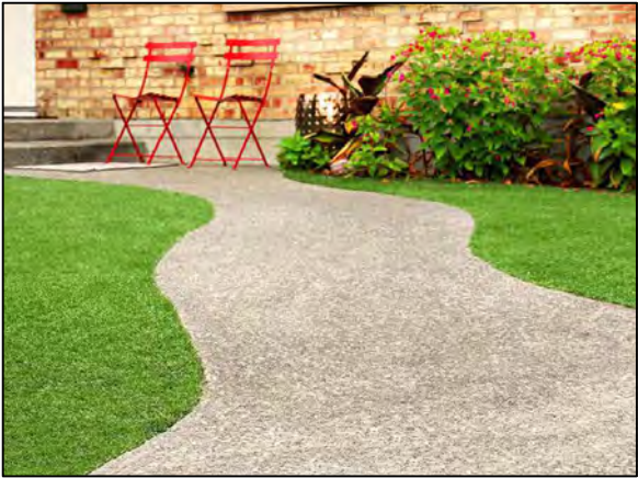
① STONE DUST WALKWAY FLUSH WITH LAWN
