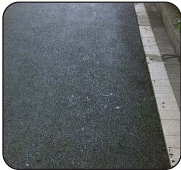
ASPHALT PAVING W/ BORDER Border Product: Prest Pavers Manufacturer: Hanover Pavers Notes: Natural Color
